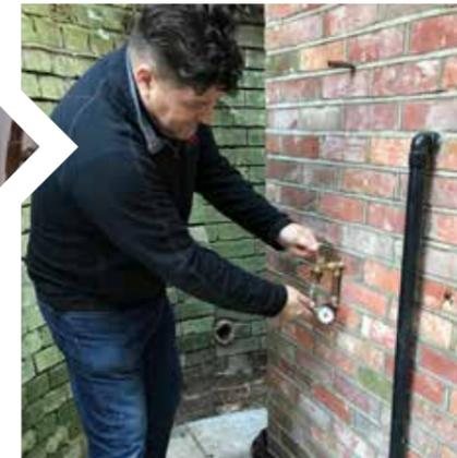
**02** Undertake a water pressure test to prevent damage/failure to the softener unit as a result of too lower/higher water pressure
