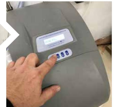
**06** Follow the easy to use settings to set the correct water softener hardness level and time using the electronic controller
