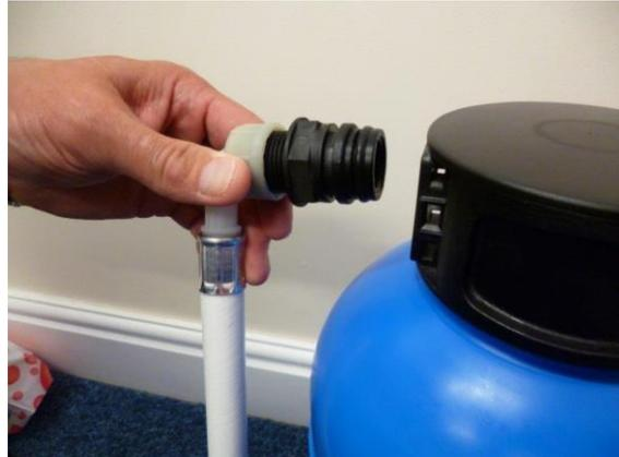
12. Disconnect outlet hose from appliance and run water from outlet hose to drain to rinse resin as per original instructions, namely;
